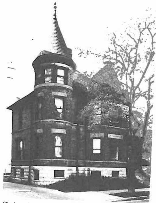
Christopher H. Starke-Charles and Matilda Baerwald House, 1327 W. Kilbourn Ave., 1897. Most Kilbourn Ave. residences were built in the 1880s and 1890s. The largest of the period are concentrated in the 1300 and 1400 blocks. Originally the homes of business executives and merchants of primarily German origin, the architecture is eclectic. Queen Anne and Romanesque styles are interspersed with houses influenced by German and Flemish architecture.
